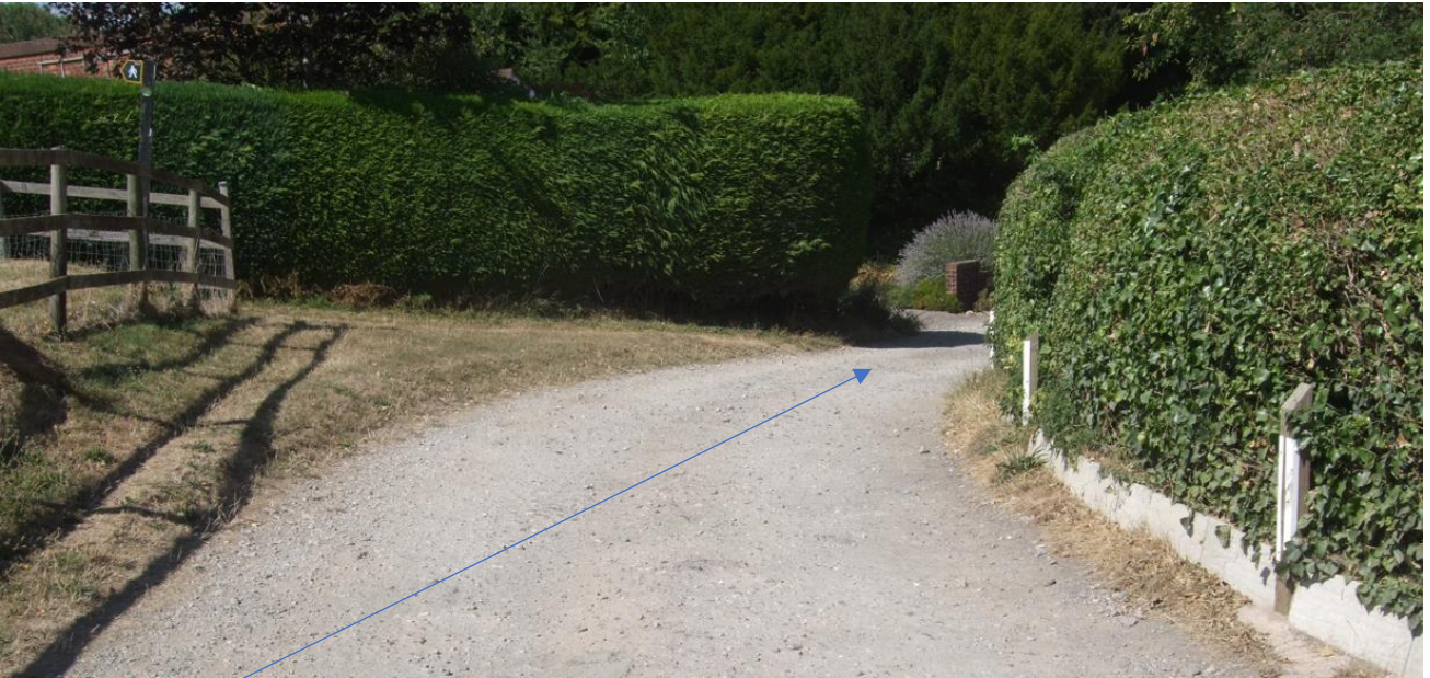
To northern end (junction with The Street)
